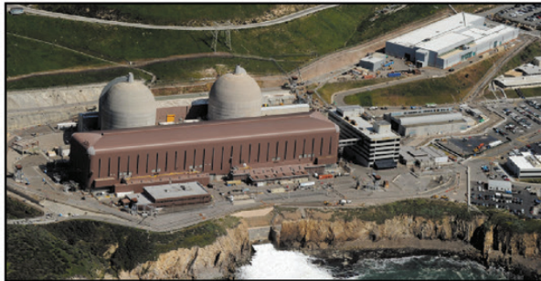
PG&E Diablo Canyon Nuclear Power Plant Avila Beach, California Required protection of a hazardous waste warehouse floor. Specified by and applied by Diablo Canyon staff, 2012.
