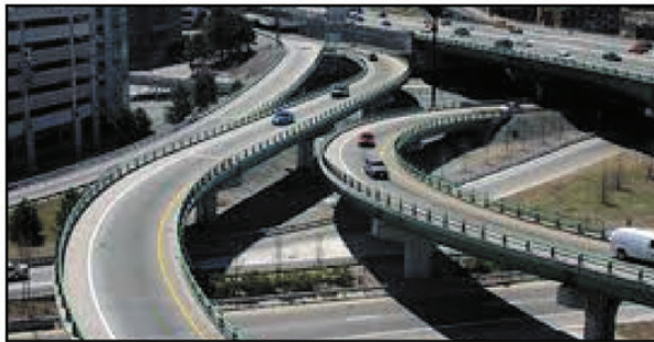
Interchanges & Causeways in Viet Nam By Obayashi Construction Co & Others 10 Million Square Feet of Crystal-Lok® applied to bridges interchanges and causeways by Vipexim, J.S.C., Hanoi
